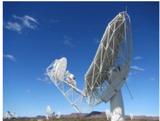
One of the 64 antennas in the telescope MeerKAT in the Karoo Desert in South Africa, with a Band 1 receiver installed. Photo: SARAO
